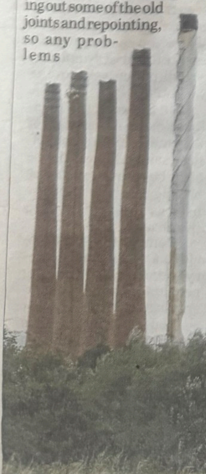
How the chimneys, left, look to passing motorists.
