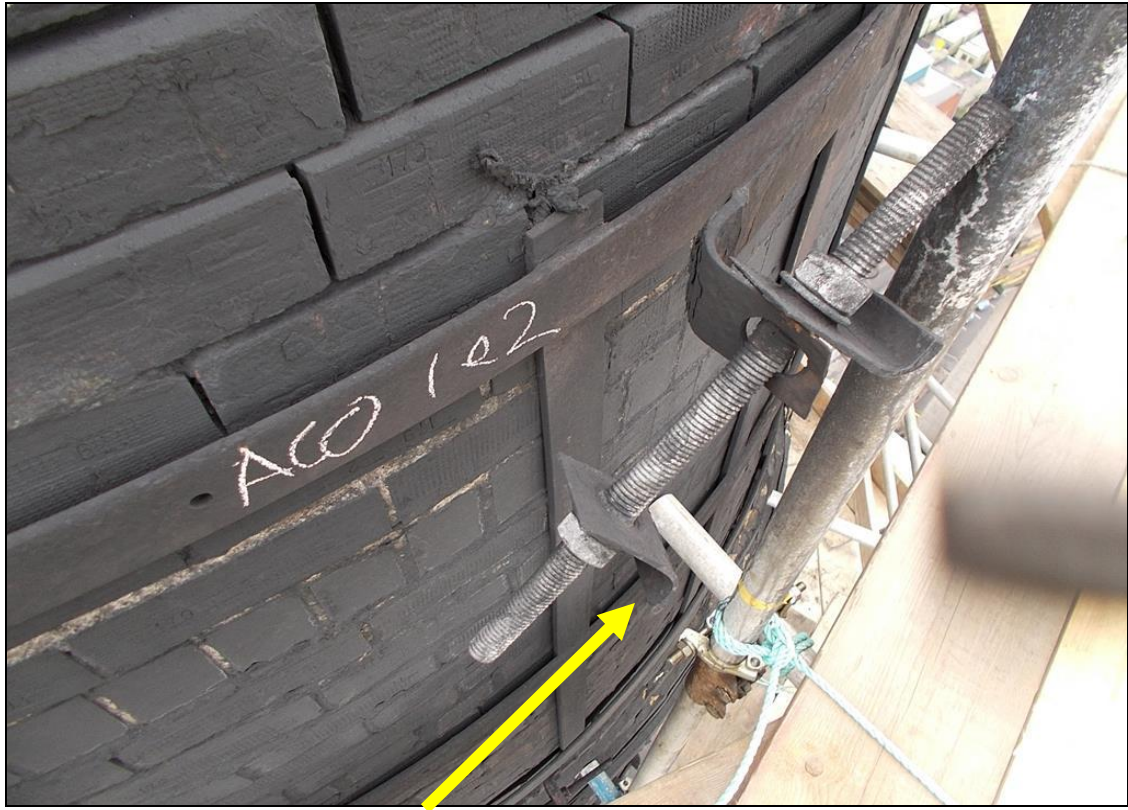
Location where the band had failed
