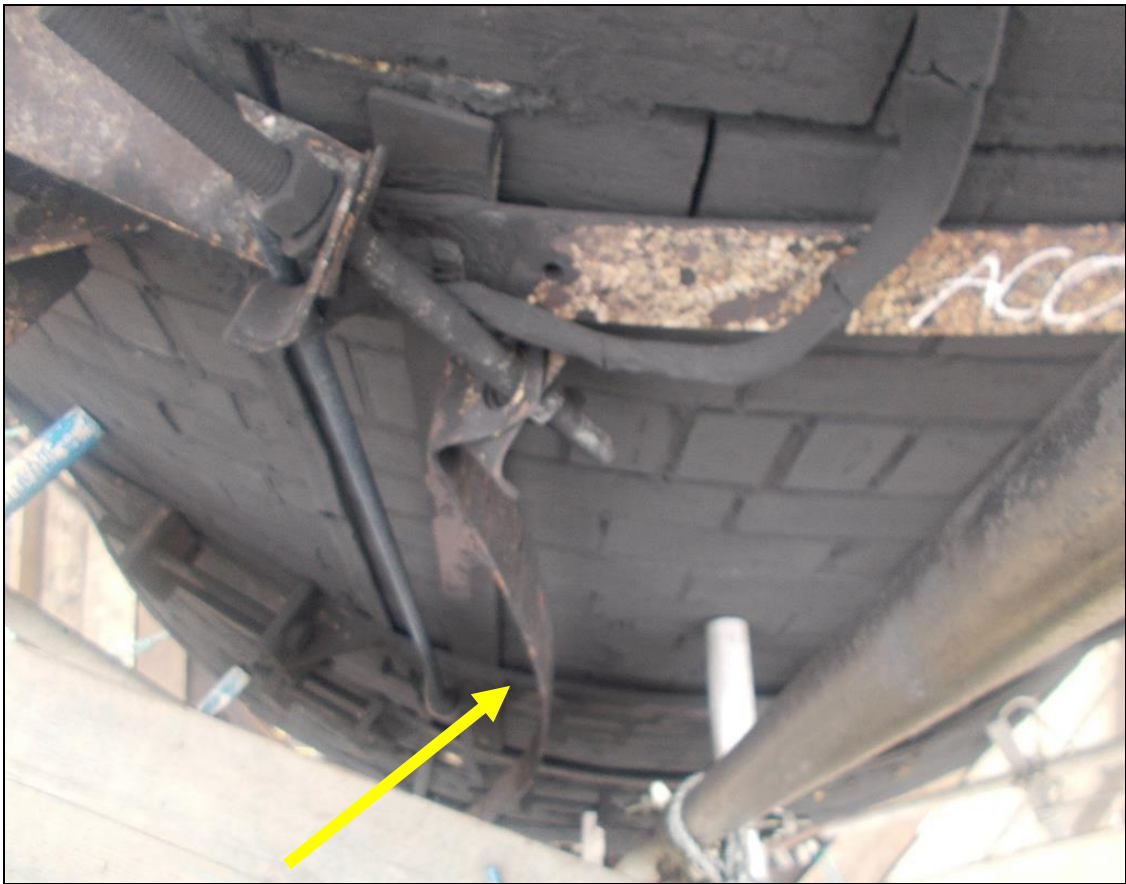
Section of the band left hanging
