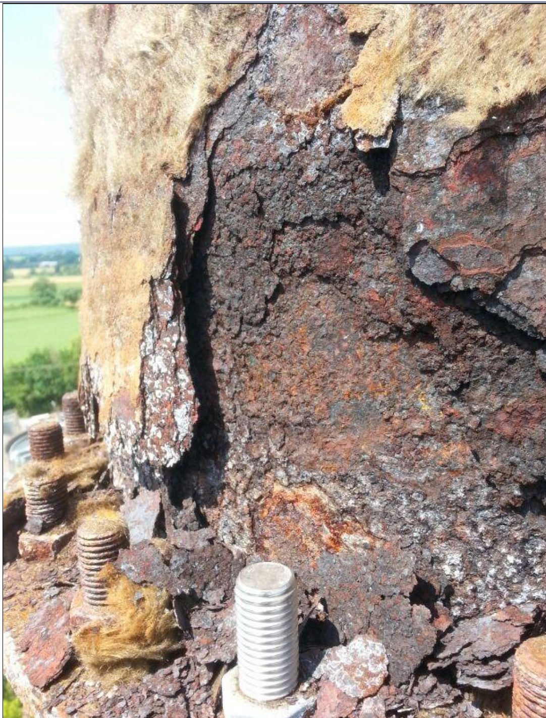
Advanced corrosion at the top flange – structural walls were found to be paper thin.
