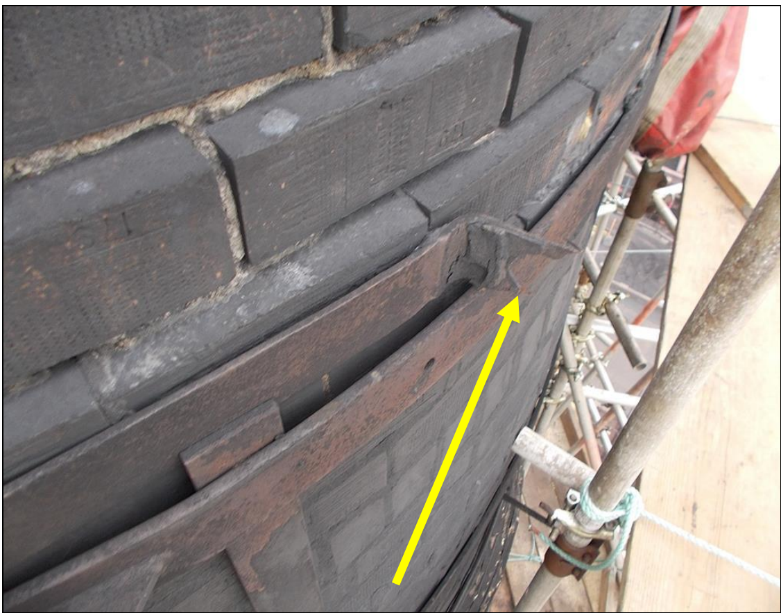
Section of the failed band stuck behind other steel work
