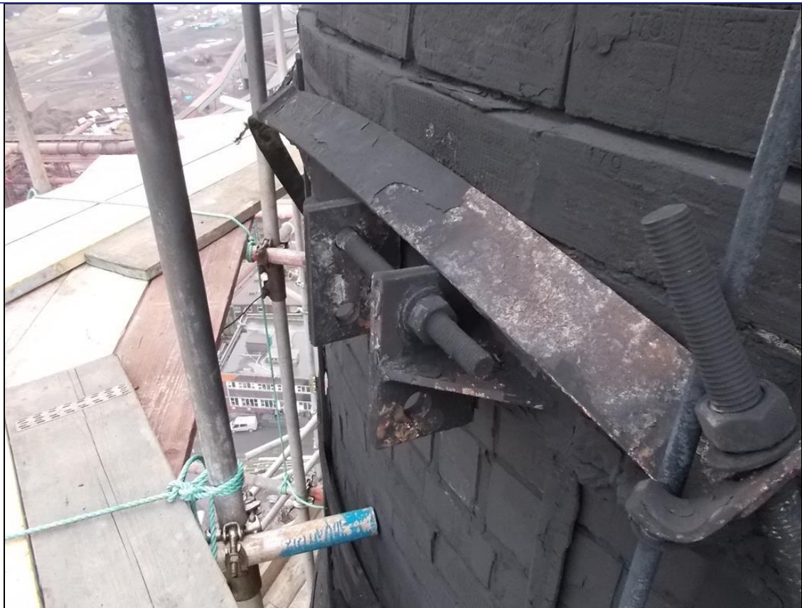
Sections of the band lodged behind a lightning conductor air terminal
