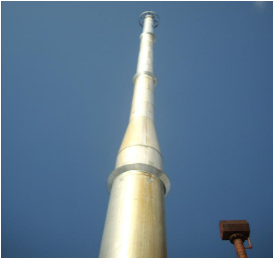
The 36.0m tall chimney prior to the inspection - fully clad and insulated
